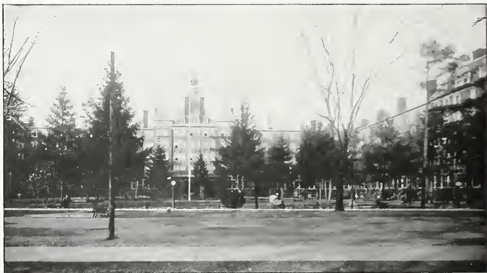
FIG. 173.—General Hospital No. 9, Lakewood, N. J.
